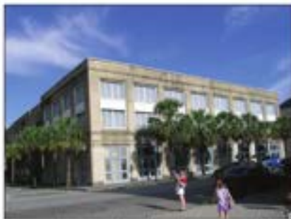
Structured parking with retail on the first floor and better screened parking level above.
