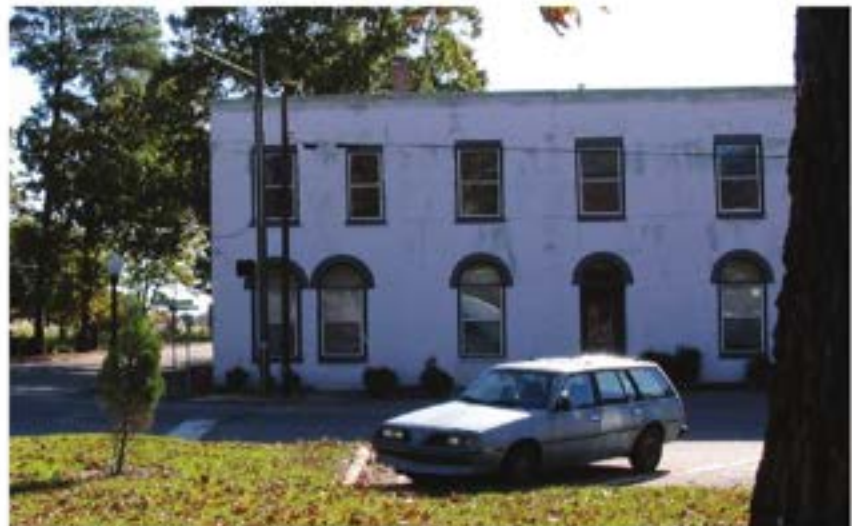
This side facade shows an appropriate window pattern and a side entry.
