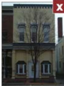
Examples of inappropriate storefront illustrations. From left to right: new storefront features a "colonial theme" that is stylistically inappropriate; reflective glass prohibits pedestrian interaction with the storefront; storefront has been removed entirely and covered up with incompatible wall material and columns appear undersized and "weak."
