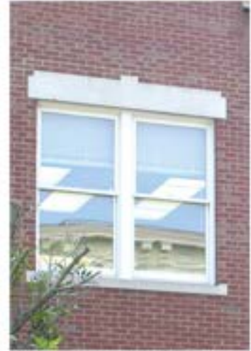
A window with projecting lintel and sills.
