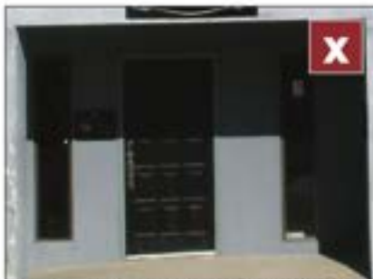
The material, detailing, and lack of transparency in these doors are inappropriate replacement solutions.
