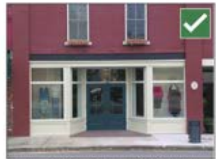
Good example of storefront renovation utilizing new materials adhering to traditional storefront composition.
