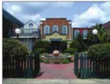
Good example of rear entrance to a commercial building with primary entrance on the street side.
