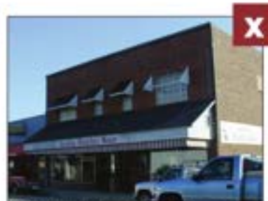
Striped canopy appears as oversized awning concealing transom, sign panel & upper facade components.
