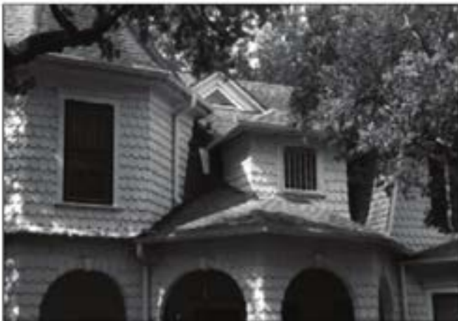
The distinctive wood shingle walls of this house on Hayne Avenue are a characteristic of the Shingle style.
