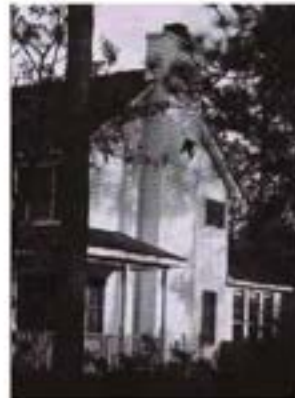
Above: Chimneys covered with vinyl siding are not appropriate for houses attempting to blend with Aiken's historic buildings.
