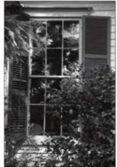
Before the English invention of machine-rolled glass in 1832, available manufacturing techniques limited window panes to small sizes. Glass was a luxury in early America, and most of it was imported until well into the 1800s. Although it was possible by the late 1800s to use a single large sheet of clear glass, the examples on the left illustrate the popularity of using glass panes for decorative effect and the revival of interest in stained glass.
