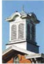
Traditional roof structures such as these cupolas can be used to house roof top equipment on gabled roof forms. On flat roofs with parapets, equipment can be placed out of site by keeping the parapet higher than the equipment.
