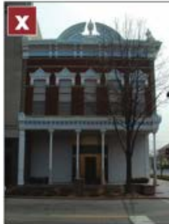
The absence of framing piers and their replacement with visually inappropriate sized columns make the building look as though it will collapse on itself.
