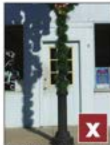
The detailing of this door is inappropriate to the building itself and the overall character of the district.
