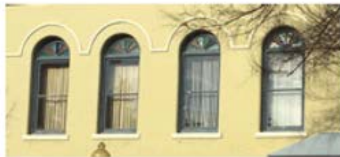
Examples of appropriate features and alignment of upper floor openings in Downtown Aiken
