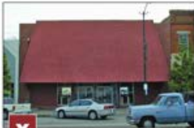
The roof form becomes the dominant element of this facade and is incompatible with its surroundings.
