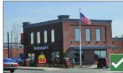
This franchise architecture (which is typically one-story tall) utilizes a false upper façade to give it the appearance of being two-stories tall in order to relate to its surroundings.
