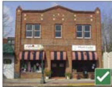
The triangular treatment at the center of the roof creates interest and delineates entry. The upper floor details such as precast tiles and recessed panels above the windows creates interest at the second floor.
