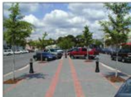
A common palette of streetscape elements such as paving, tree plantings, bollards, vintage light poles, and clearly demarcated crosswalks create both an attractive and safe downtown.
