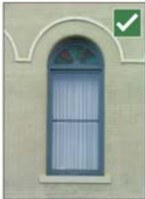
This arched-top window appropriately fills in the entire masonry opening.
