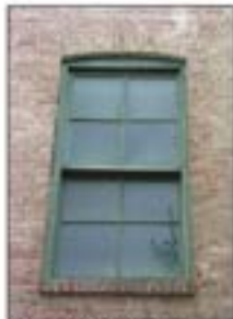
True divided light wood windows were the norm in traditional construction. 4-over-4 pattern.
