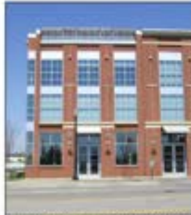
Successful "contemporary interpretation" of the traditional storefront separating the "display windows" with brick piers, and maintaining recessed door entry.
