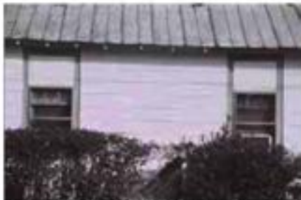
Although the original windows appear to be still intact in the example above, ill-sized storm windows have been placed over them. The gaps created by the too-small storm windows have been filled in with wood at the top, greatly compromising the appearance of the windows.
