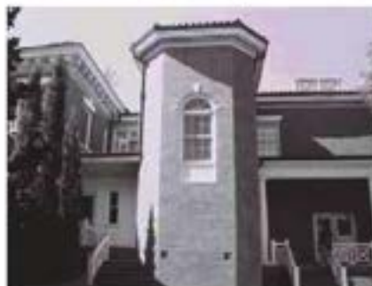
Built in the early 1900s, this residence was enlarged considerably for use as a hotel. Both rear and side additions were made for the new use. While the brick and roofing of the additions match that of the old structure, the detailing is less elaborate. The form of the original house, which is still dominant, is evident.
