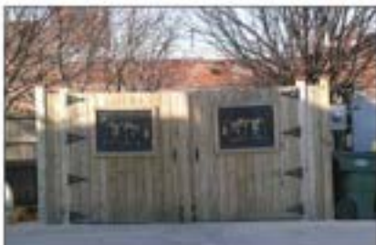
Good example of screening service equipment and trash bins utilizing wood gates with wrought iron ornament.
