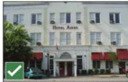
Long building sub-divided into bays with clear hierarchy and delineation of entry.
