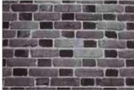
A brick bond, such as this Flemish bond, can be an important design feature.
