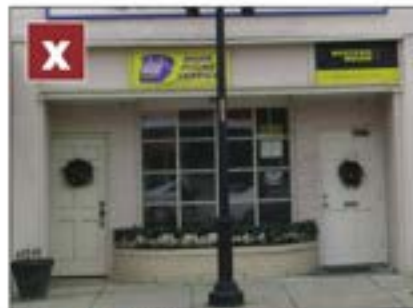
The material, detailing, and lack of transparency in these doors are inappropriate replacement solutions.
