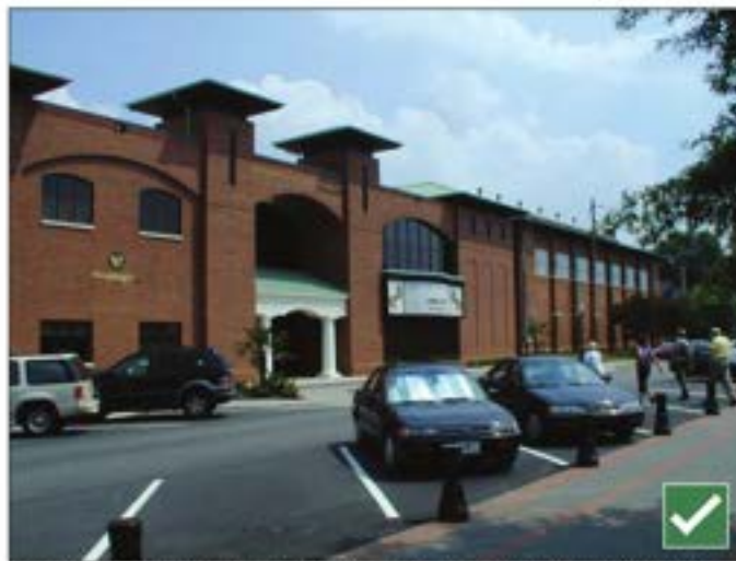
Good use of brick as the predominant building material on a new building. This choice of wall material not only relates to the adjacent Court Tennis building, but also the downtown area as a whole.
