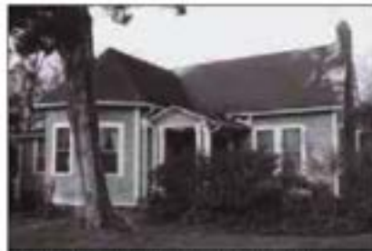
The downspouts of the house above are correctly positioned on porch supports and at the corners of the building.
