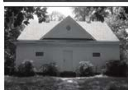
Enclosure of a front porch will not normally be allowed by the Review Board because it can dramatically alter the appearance of a house. The two houses in the above photographs, which are next door to each other, were probably once almost identical.
