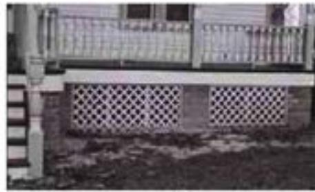
Lattice is an appropriate infill between piers, especially for porches. It allows air circulation to prevent moisture from accumulating under a building.
