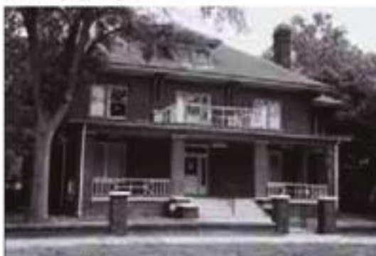
The use of a different or contrasting color can make a feature stand out—as with the white railings on this building.
