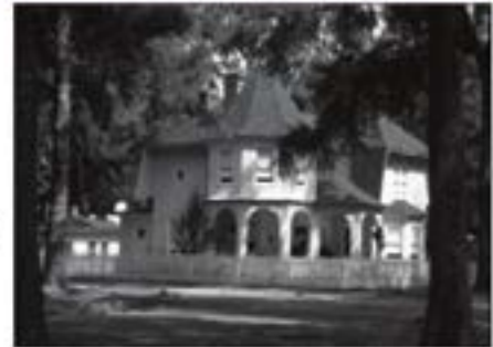
The complex roof shape and tower of the Charlie Hill House (303 Newberry Street, NW) are important to the design of the Shingle style house.
