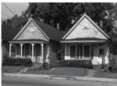
Above: The detailing of the porch on the right probably was once the same as that of the house on the left. The metal supports are inappropriate because they completely alter the character of the porch.
