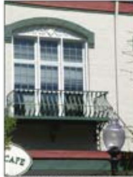
Well executed balcony and support bracket.
