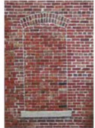
A bricked-in opening or "blank" is an appropriate method for continuing a window placement pattern in areas where interior layouts do not allow for true openings.
