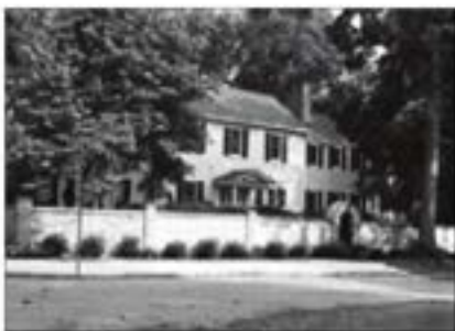
The aluminum siding on Rest Period (above) was painted because its finish had worn.
