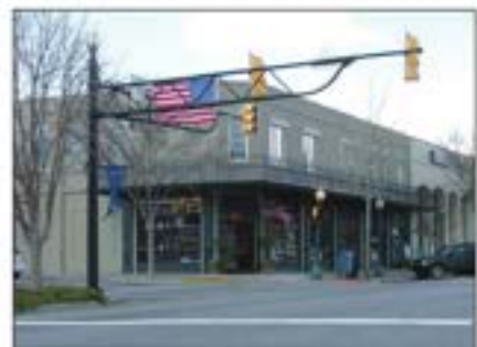
A common palette of streetscape elements such as mast arm traffic signals, tree plantings, vintage lights, benches, and clearly demarcated crosswalks create both an attractive and safe downtown.
