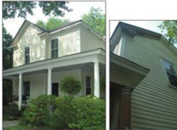
Above: The renovations on this house included removal of synthetic siding. Because the synthetic siding did not have the same dimensions as the original wood siding, it had significantly altered the appearance of the building.
