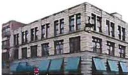
This design is far more appropriate due to its continuous horizontal trim and recessed windows, as well as the creation of bays at the first level.
