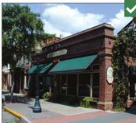
Perfectly executed awning installation.
