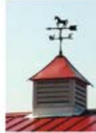
Traditional roof structures such as these cupolas can be used to house roof top equipment on gabled roof forms. On flat roofs with parapets, equipment can be placed out of site by keeping the parapet higher than the equipment.
