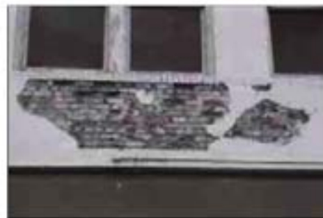
Covering masonry with another material to mask symptoms of moisture accumulation will not be allowed. Measures should be taken to deal with the problem rather than to hide it.
