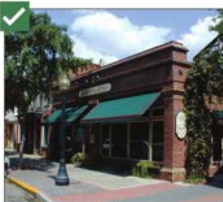
Perfectly executed awning installation.
