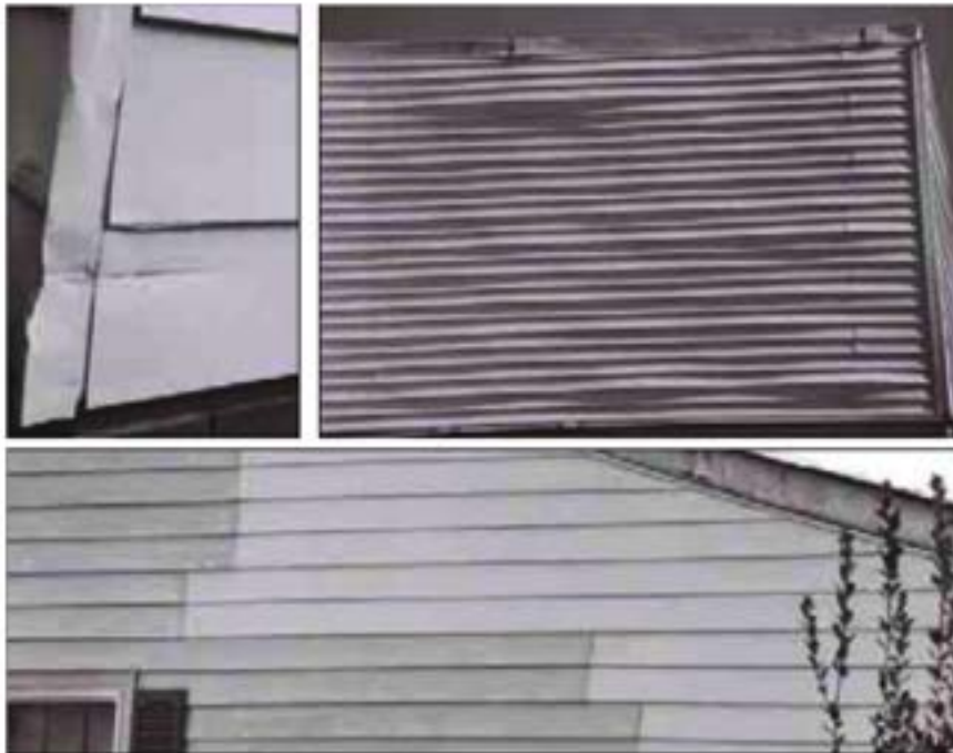
Some disadvantages of synthetic siding include dents from impact on aluminum (top left); permanent distortion of vinyl caused by exposure to temperature extremes (top right); and the difficulty of matching colors, which can change over time (above).
