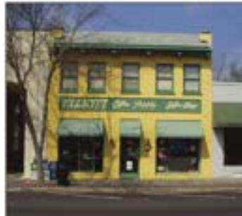
The piers on this building are expressed clearly by virtue of their material, color, and continuity from the first floor to the upper floor.
