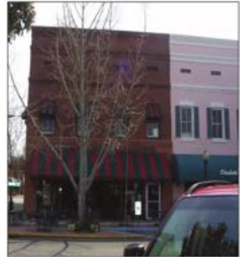
These two buildings do a good job of expressing the masonry piers that support the upper façade. However, they could have been improved had the awnings been constrained within the piers.
