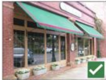
The preservation of the existing brick on this building relates it to the entire downtown area.
