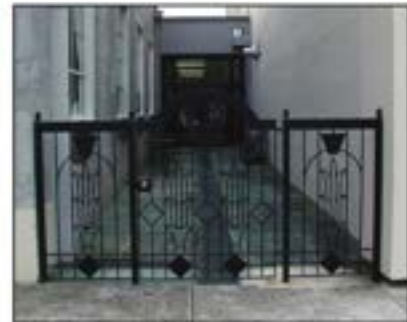
Ornate wrought iron gate segregating an alley entryway from the public sidewalk.
