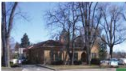
This fast-food restaurant uses a gabled and hipped roof form, this roof type is appropriate on commercial-type buildings less than 15 feet in height in neighborhoods.
