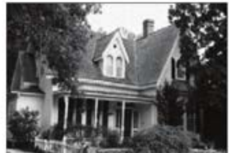
A new wood shingle roof was installed on 320 Fairfield Street, SE, in the mid-1990s. The installation matched as closely as possible an old wood shingle roof found under asphalt roofing shingles. The old wood shingles had a green tint, which probably was a chemical treatment for inhibiting the growth of fungus.
