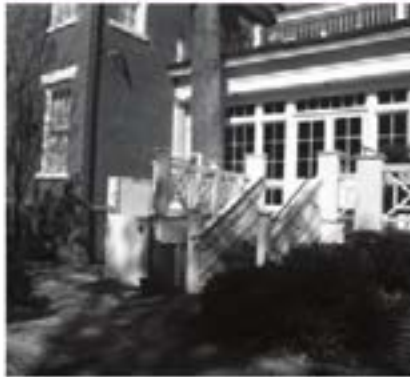
Above left: The wheelchair lift at Woodlands in Summerville provides access near the front entrance and eliminated the need for a ramp. Such lifts are effective for three-to-ten foot changes in elevation.
