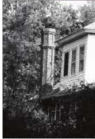
The octagonal chimneys of Rose Roof were constructed in the 1920s and are unusual in this area. They could have been inspired by chimneys from the native lands of Elise and Frederick S. Wilcox, who were from Europe.
