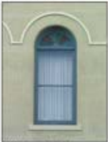
Arch-topped windows can provide visual interest and character to a building. 1-over-1 pattern.
