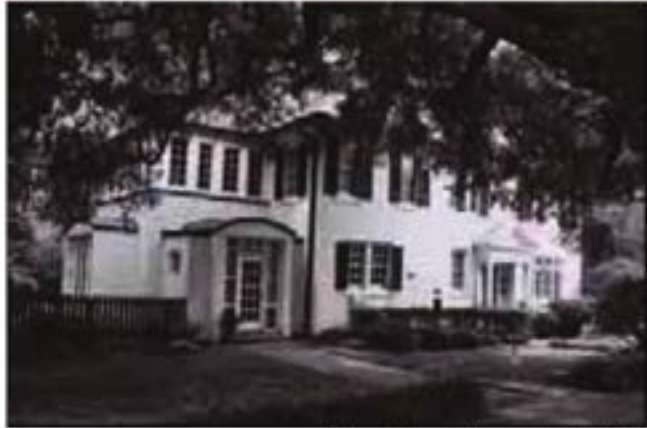
Above: The small, one-story additions on the left do not detract from the original design of the house.
