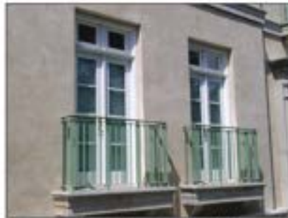
Contemporary interpretation of traditional balcony element creates a sense of extending the inside of the building to the outside.
