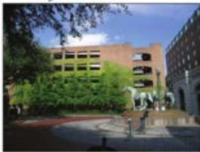
Heavily landscaped structured parking to conceal utilitarian use. Use of quality building material such as brick.
