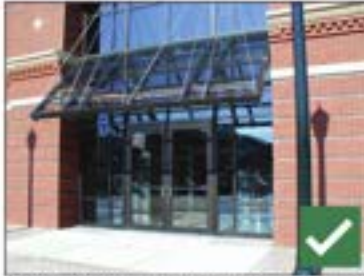
Metal and glass canopy interprets the historic role of a canvas awning or metal canopy and clarifies entry on this new building.
